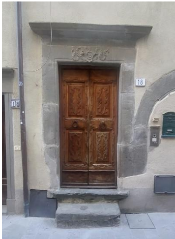
16 Door with decorated architrave at number 18
